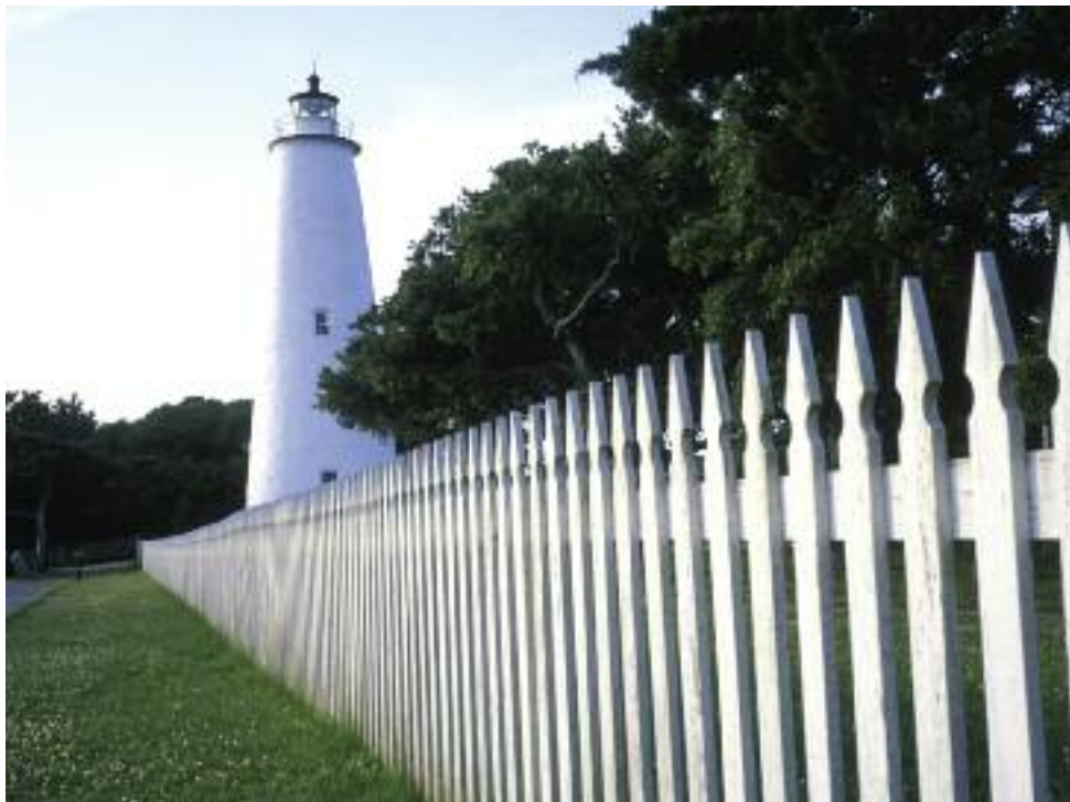
The second oldest operating lighthouse in North Carolina, the Ocracoke Lighthouse is open to the public for tours.
